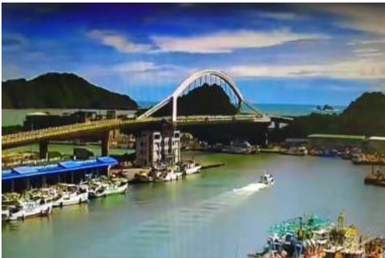
The Nanfang'ao Bridge collapsed in Taiwan (2019)
