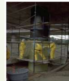
Fiberglass & Epoxy Composite Jacket
