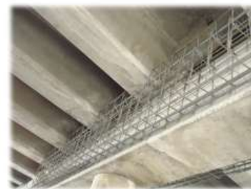
Bolster Reinforcing Steel
